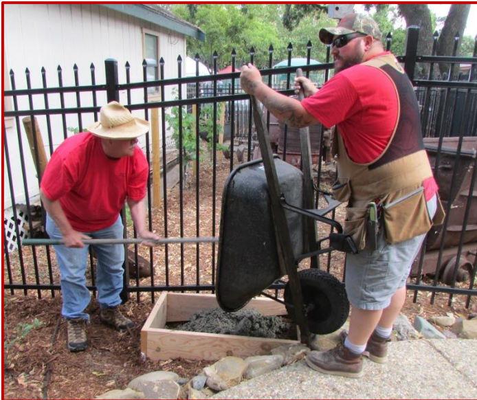
Eric Sorensen (L) and Jason Arthur (R) pour the first load of concrete for the monument base.
